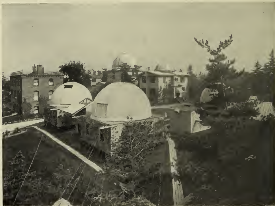
OBSERVATORY BUILDING FROM THE NORTH
